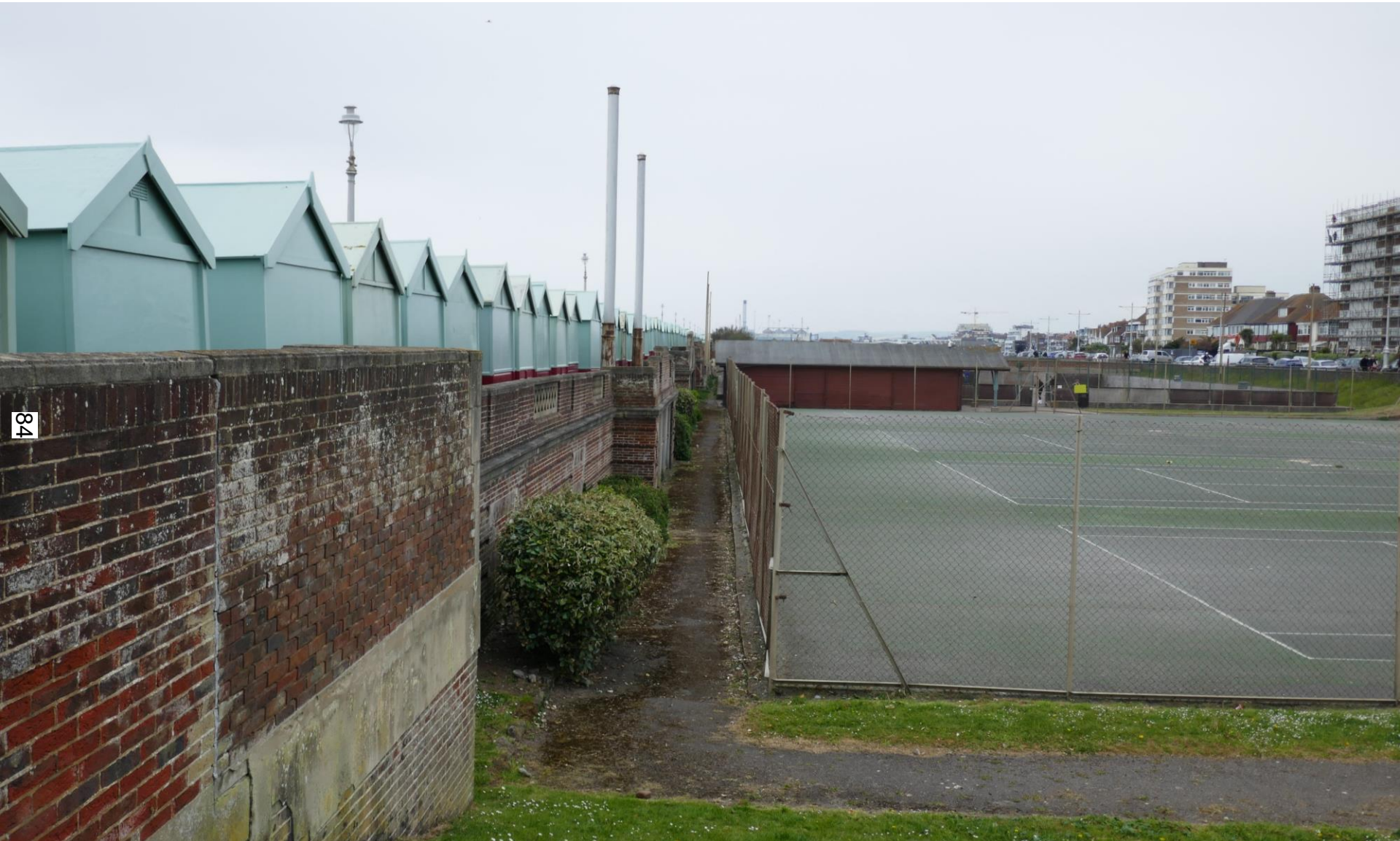
Existing View beside Tennis Courts, looking west
